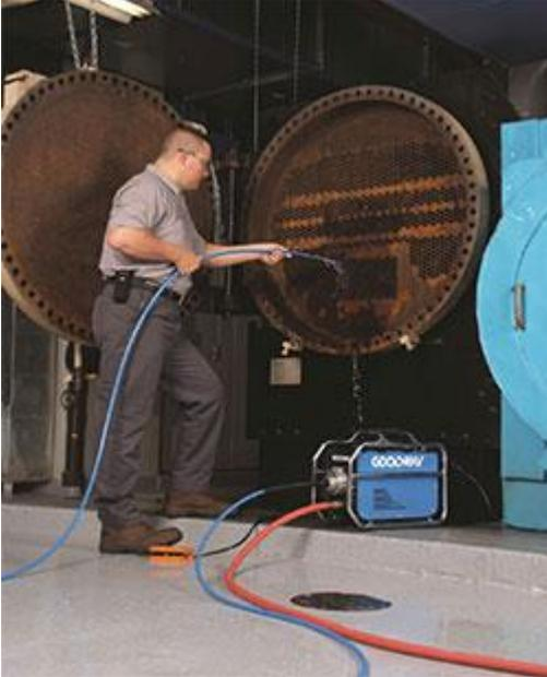
**There is a variety of chiller tube cleaning equipment and accessories that are simple to use, portable, and can be easily operated by one person.**
